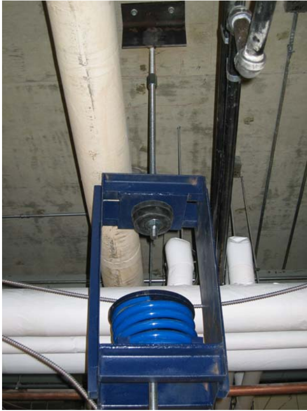
Figure 9: Isolation hanger at front of inertia base.
