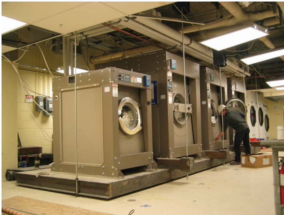
Figure 11: Inertia base during installation.
